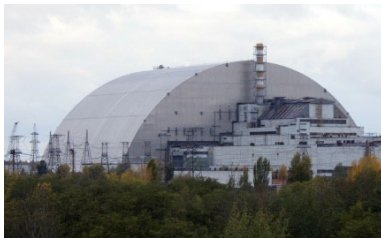
Destroyed reactor 4 building – it is now covered under a sarcophagus structure as well as the recent new safe confinement, the biggest moving structure on Earth [16]
